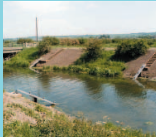
Measurement of river flow for abstraction control and flood prediction. This is an example of transducers in crossed path configuration, mounted on sloping racks.
