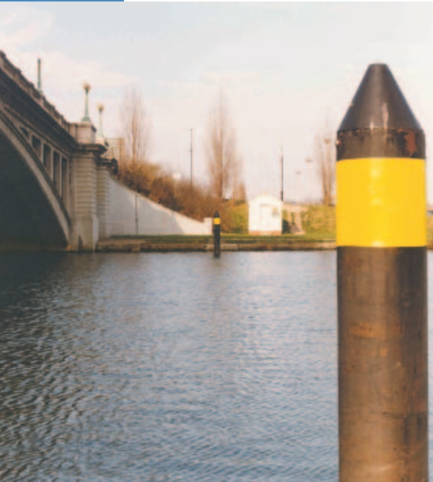
Measurement of river flow for abstraction control. This is an example of transducers in crossed path configuration, mounted in round steel piles for protection from navigation.
